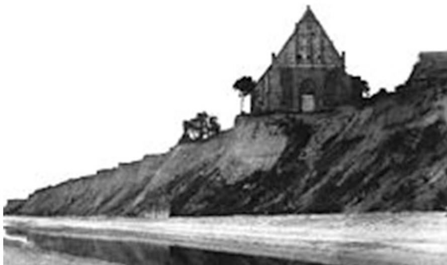
**Fig. 6.15** Location of the historical church in Trzęsacz in 1870 (Sarosiek 1972). Since the inception of the church and the village, the cliff coast retreated 2 km to the south. Erosion processes have occurred here in the area of glacial moraine
