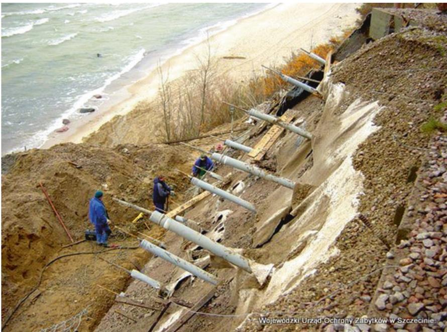
**Fig. 6.18** Protection works on the cliff supporting the Trzęsacz church; installation of oblique ground anchors (Source: <http://wybrzeze-rewalskie.pl/atraccje/ruiny.html>)
