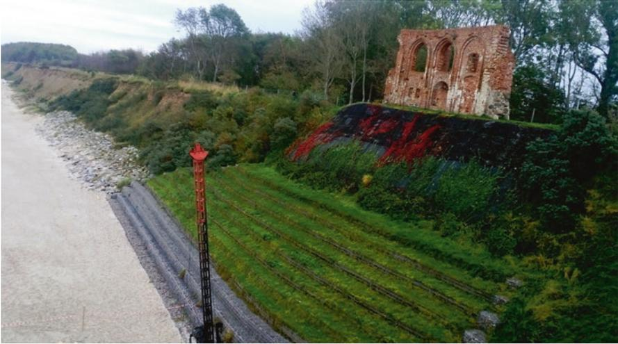
**Fig. 6.19** Gabion- and Green Terramesh-protected cliff with ruins of the southern wall of the Trzęsacz church (summer 2014)
