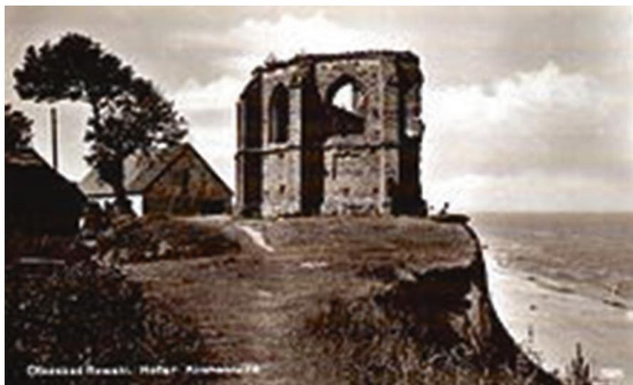
**Fig. 6.16** Fragments of the Trzęsacz church, with the missing northern wall, in 1930 (Sarosiek 1972) after a further 60 years destroying of the sea shore
