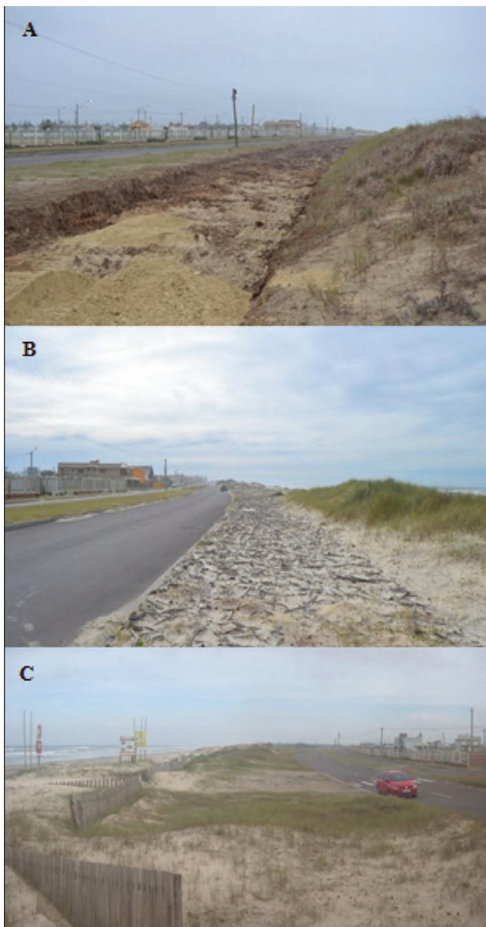
**Fig. 3.3** Planned retreat of the road. (a) Removal of the residues from the old road; (b) placement of bark fragments; (c) restoration of the natural system, with vegetal cover
