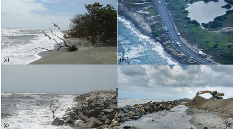
**Fig. 23.4** Examples of coastal erosion and flooding along the study area. (a) and (b) Erosion at Kms 18–19 during 2014, (c) and (d) revetment building in order to mitigate coastal erosion and flooding. Photo b: El Heraldó
